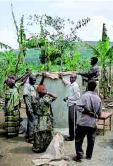
Tank construction as training.
